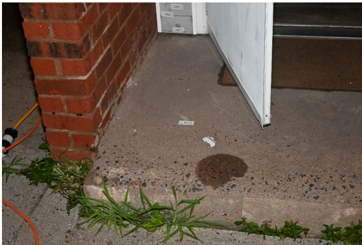
[Bullet defect in concrete front stoop]
